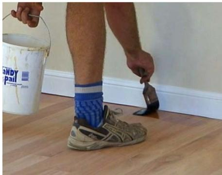
Do the cutting in first, because this will let you walk around on the body of the floor. Use a clean, good quality brush to cut in around the perimeter walls and in difficult to access places.
