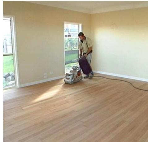
The number of passes required, and the grades of sandpaper used to complete each stage, will depend on the condition of the floor and the hardness of the timber species.
