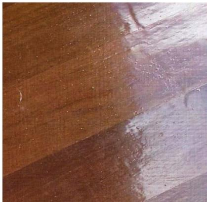
There are lots of contaminants that can float in the room and settle on the floor while it's drying. They include dust particles, hair, insects and grit.
