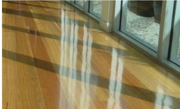
Some systems take up to two weeks to fully harden. Although the floor can be walked on after the initial drying period, it is much more prone to scratching and scuffing until it is fully cured. So although the client might want to rush in and put their furniture in place, you should advise them to be very careful until the manufacturer's recommended waiting time has elapsed.
