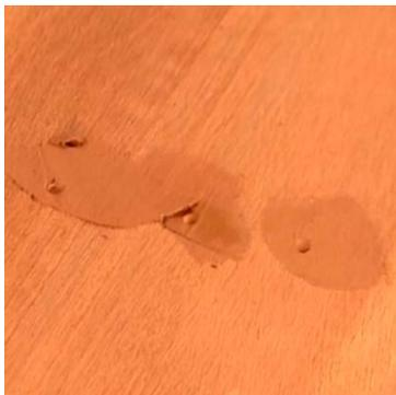
Some contractors like to fill the nail holes before they sand the floor, so that the filler is sanded flush as part of the overall process.
