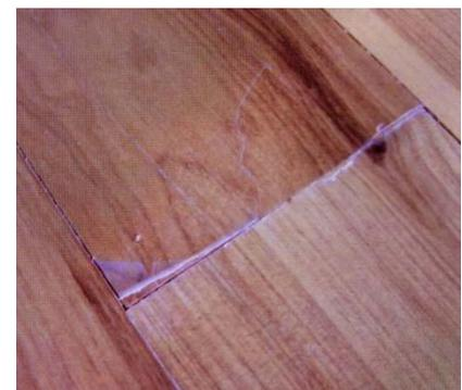
Delamination can also occur between coats if an incompatible product is put on top, or if there is insufficient keying into the previous coat. In these cases, the floor generally needs to be sanded right back to raw timber and the finishing process started again.
