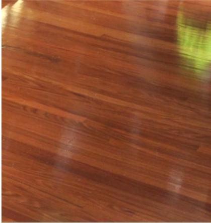
Solvent-based polyurethanes sometimes show variations in gloss levels. This can happen if the base coat wasn't sufficiently cured or sanded to a uniform finish prior to the final coat being applied.
