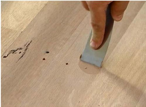
Any nail holes and cracks that haven't already filled should be filled, or 'stopped', once the first coat is dry. Use a clean-bladed putty knife or applicator to push the filler fully into the hole.
