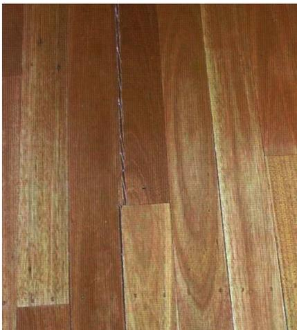
Edge bonding happens when a coating product seeps into the gaps between boards and glues them together.
